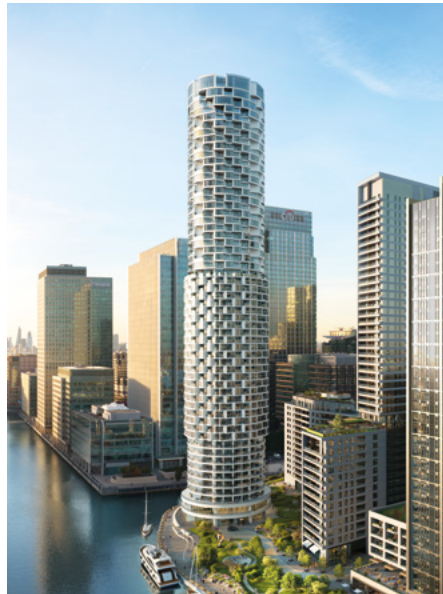
One Park Drive, Canary Wharf – Herzog & de Meuron's first residential building in the UK*
