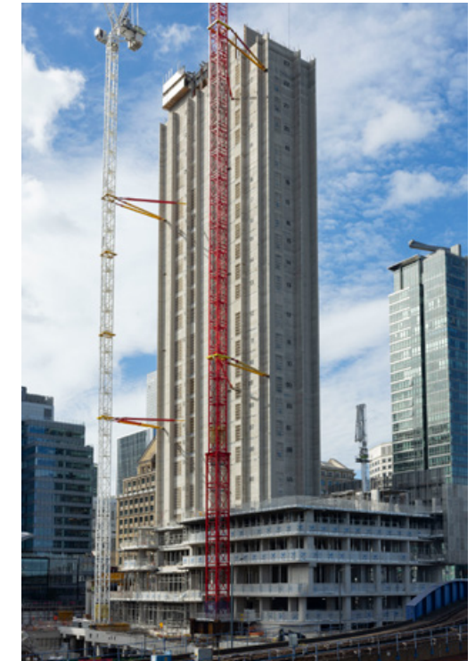
Floor slabs at level 5 on the north elevation
