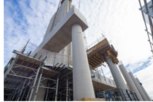
Double height marine deck columns and transfer beams
