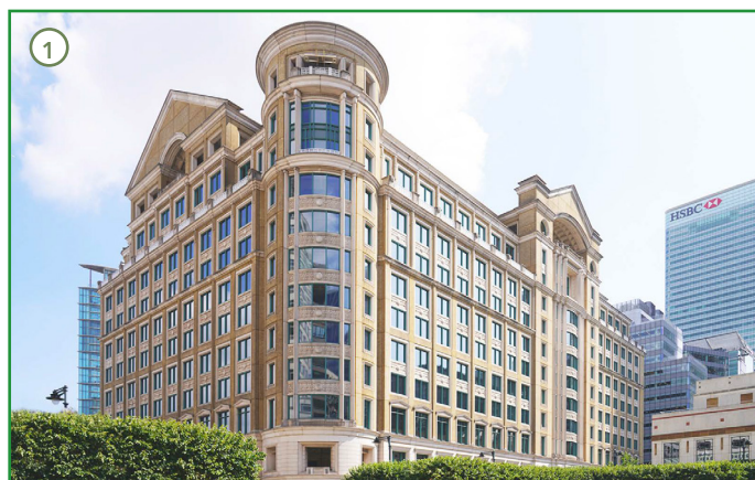
Existing building - view from south west
