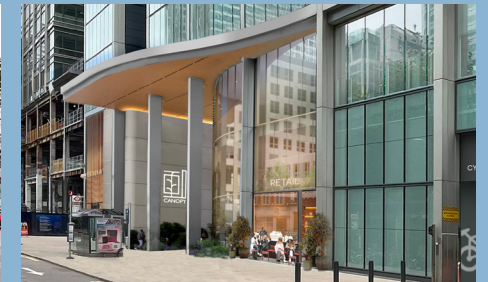
2. Retail unit adjacent to north entrance
