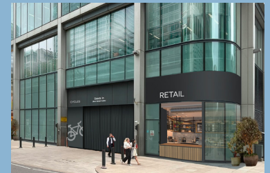
3. Retail unit, north-western corner
