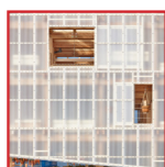
Polycarbonate cladding to foyer
