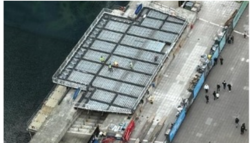
The raised terrace being installed at Middle Dock
