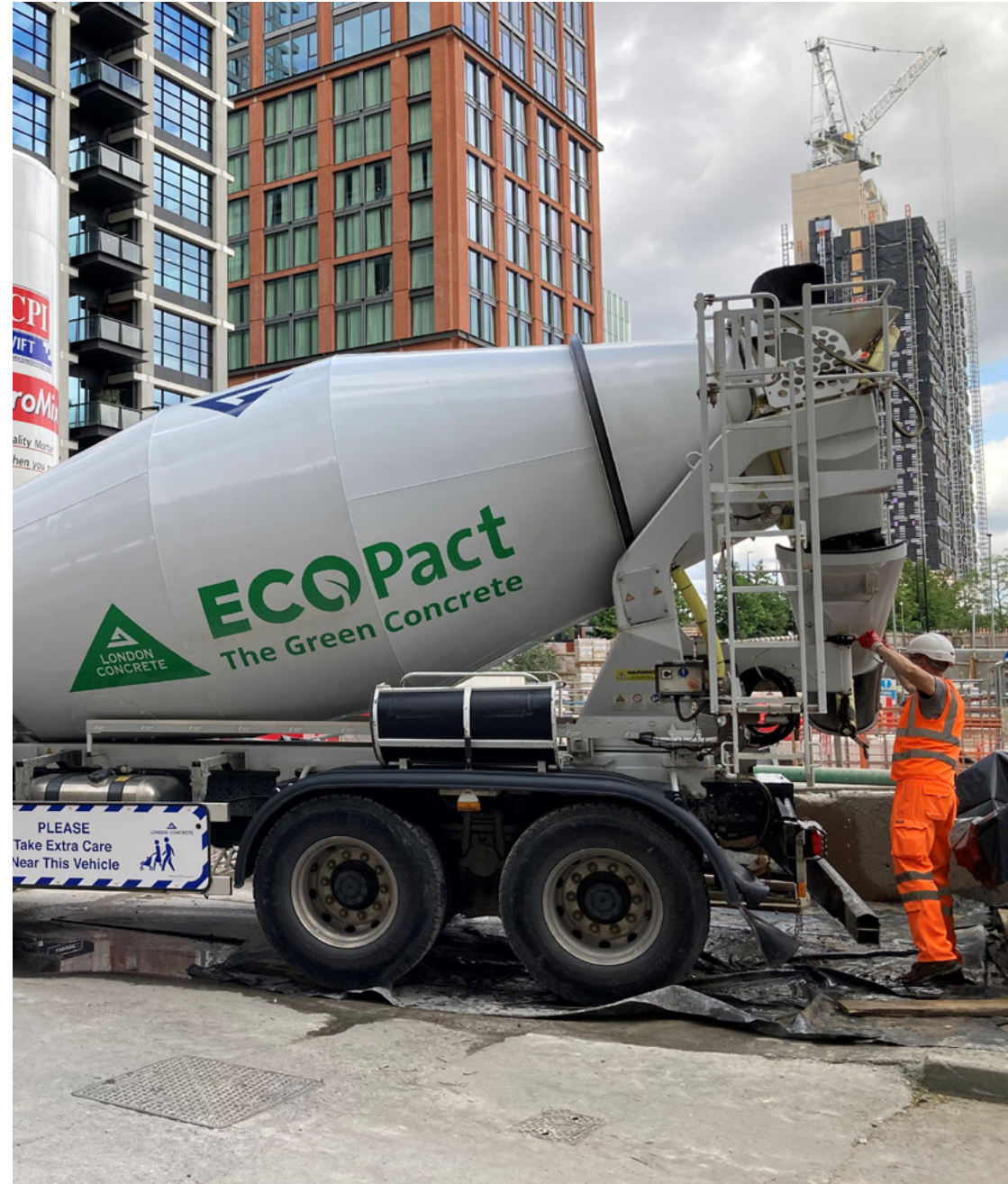
Fully electric concrete mixer at Wood Wharf
