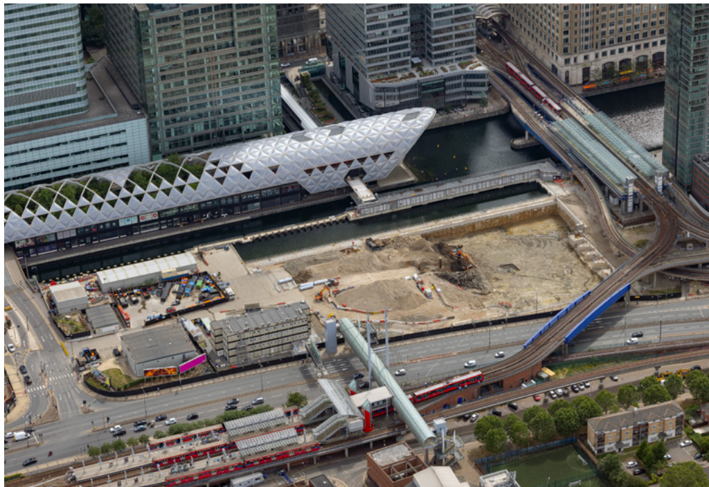
North Quay site, April 2023
